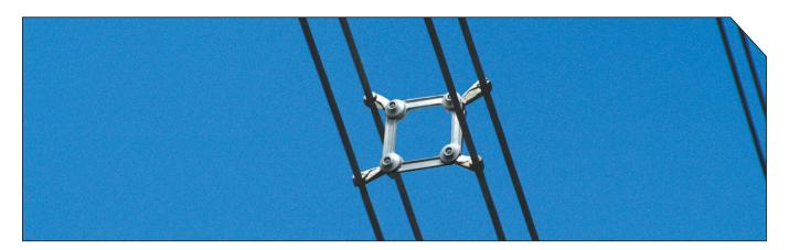
PLP's range of CUSHION-GRIP Spacer Dampers feature elostomer damping elements engineered to absorb maximum energy and protect valuable line hardware. The design provides utmost resistance to conductor fatigue and eliminates the need for additional Stockbridge type dampers. The CUSHION-GRIP range is available for twin, Tri, Quad and hex bundle configurations.
